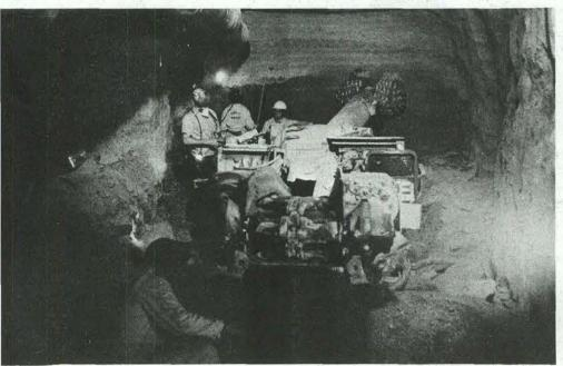
HOW a tunnel is created is shown in this photo, taken in nearby G-Tunnel. Electrically driven bits at head of this Alpine mining machine chew into soft volcanic tuff; loose material is then disgorged at tail end of machine for removal. Geologist Bill Vollendorf (1133) glances toward camera.
